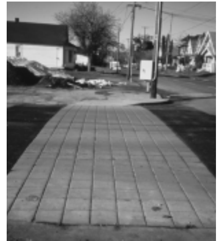
A change in paving materials at pedestrian crossings can make the crossing more visible.
